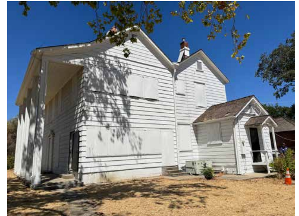
Figure 13: The east elevation of the Main House, view northwest (2024).
