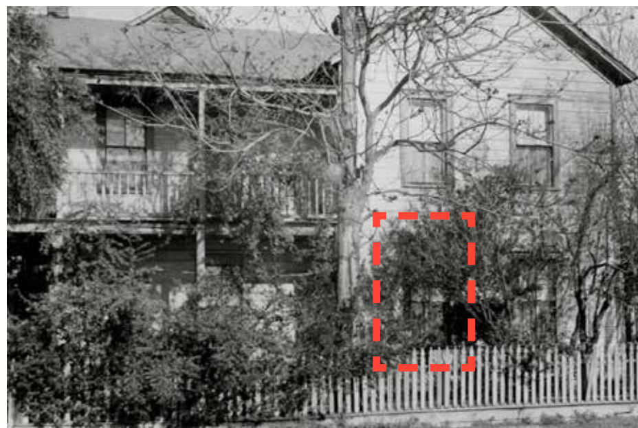
Figure 14: Photograph of the west elevation taken in the 1920s, showing the location of a window recommended to be reopened (outlined with dotted red line). Source: Roseville Historical Society.
